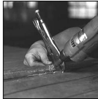
20. Now press the cleat into position and fasten with a metal screw. Install at intervals according to the following schedule:
