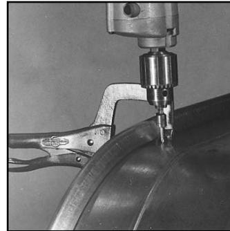
10. Work in one direction around duct when seating the frame. Fasten in sequence as you go.
