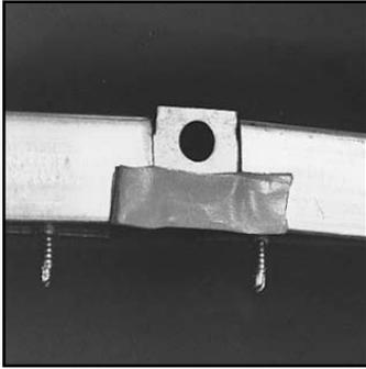
13. On all Ovalmate connector pieces apply Ductmate 440 Gasket as in photo (approx. 3"). Position 440 Gasket so that it covers the raw edge of the duct protruding past the Ovalmate connector pieces.
