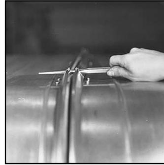
17. Align mating frames. A drift pin or Ductmate alignment grips can be used to correct any misalignment. Compress gasket with clamps.
