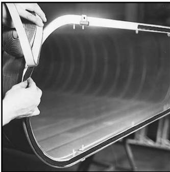
15. Press gasket firmly into contact with the face of the Ovalmate flange and the connector pieces. Ductmate Neoprene is the preferred gasket.
