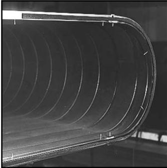
14. Start applying Ductmate Neoprene Gasket Tape to the face of the straight Ovalmate angle about halfway between connector pieces. Position gasket in the center of the Ovalmate angle as in photo. When crossing connector pieces place the gasket over the raw edge of the duct.
