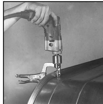
12. Continue in one direction around the duct at evenly spaced intervals as per the schedule below. Place last fastener within 1" of the end of a straight or curved flange section
